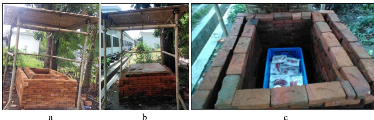
Figure 1 ZECC construction. a and b, Front side; c, Postharvest chili stored inside ZECC.
